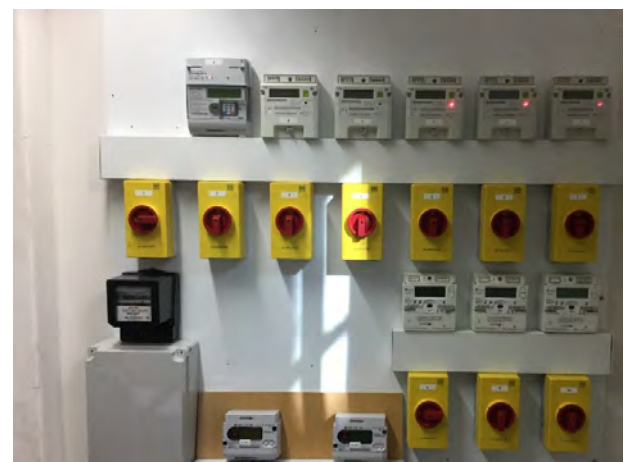
Figure 1: Smart Electricity Meters in Joule House
