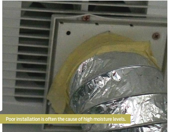
Poor installation is often the cause of high moisture levels.
